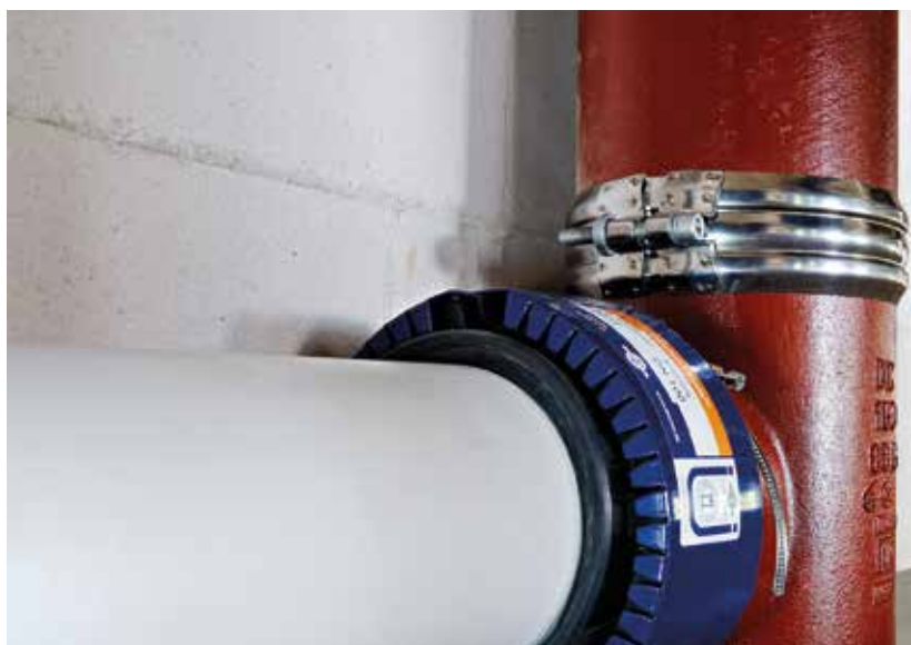
Curaflex® Konfix™ after installation at the building site
