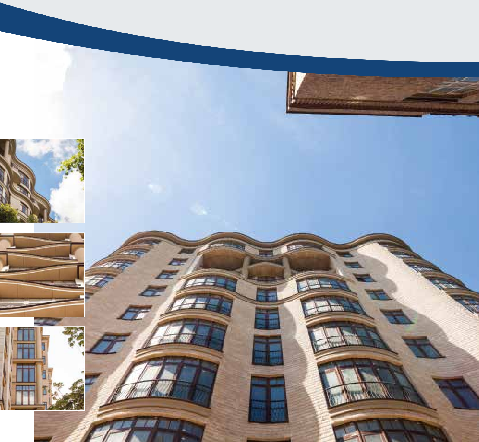
International projects Luxury housing complex in Moscow
