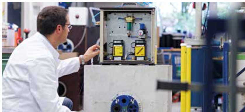
Leak test on sections of a multi-utility service entries
